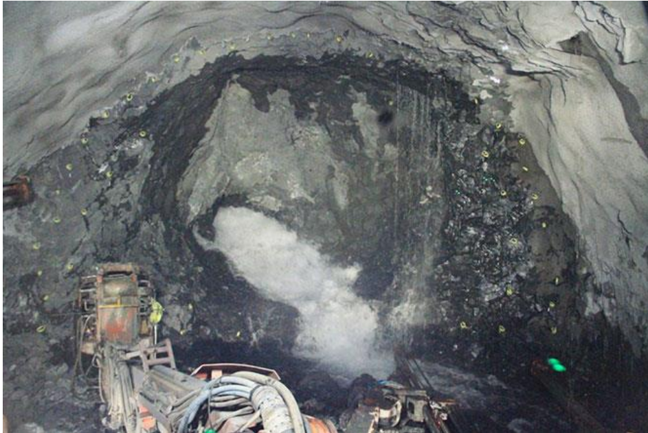
Groundwater Inflow in Fractured Rock (Example)
