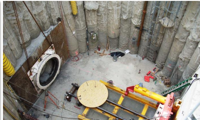
Shaft Excavation
