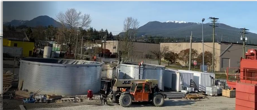
Water treatment facilities with sedimentation and pH monitoring
