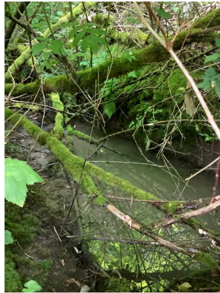
Photo 14: looking south (downstream) at the channelized drainage from the existing storm runoff at the Option 3 Outfall, from Government Road (June 10, 2021)
