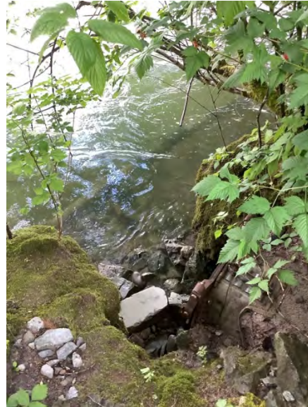
Photo 4: Looking down at existing outfall pipe and rip rap (June 12, 2021)
