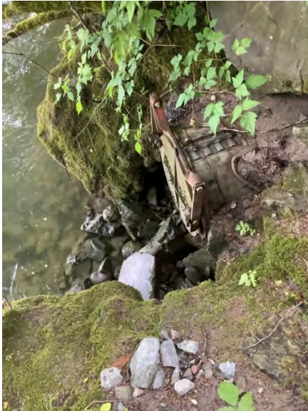
Photo 3: Looking down at existing outfall pipe and rip rap (June 12, 2021)
