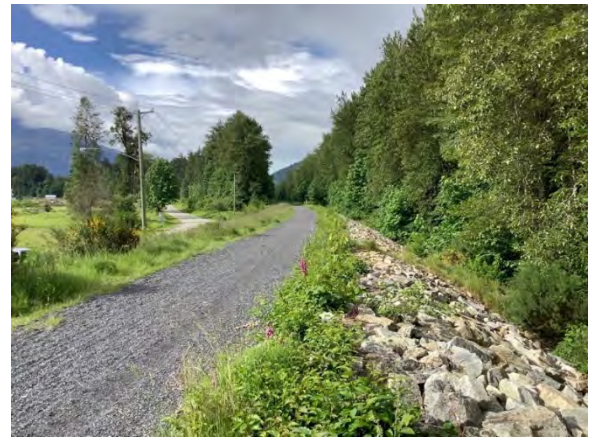
Photo 2: Looking south along the dike at the Option 1 outfall. Outfall location is to the right, through riparian band of trees (June 10, 2021)
